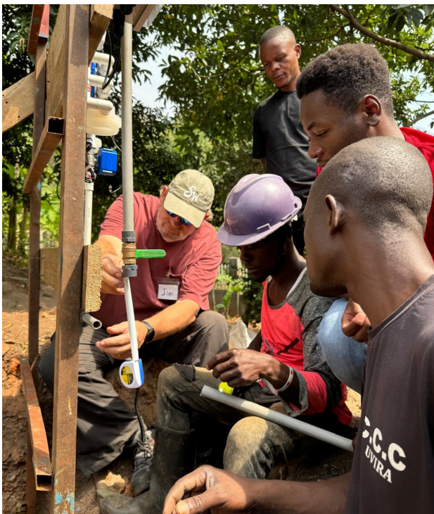
Jim and CCC staff installing water filtration system.
