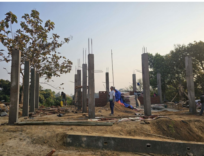
New church under construction at Kana Village
